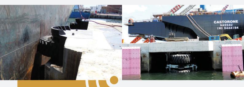
Wheel fenders are widely used on exposed corners to help ships maneuver into berths and narrow channels such as locks and dry-dock entrances.
