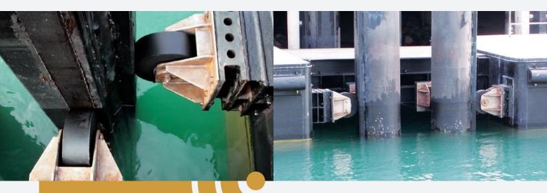
Cushion rollers are used to guide pontoons and floating structures quietly and gently up and down their guide piles.
